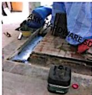
Re-surfacing of drain using W1
